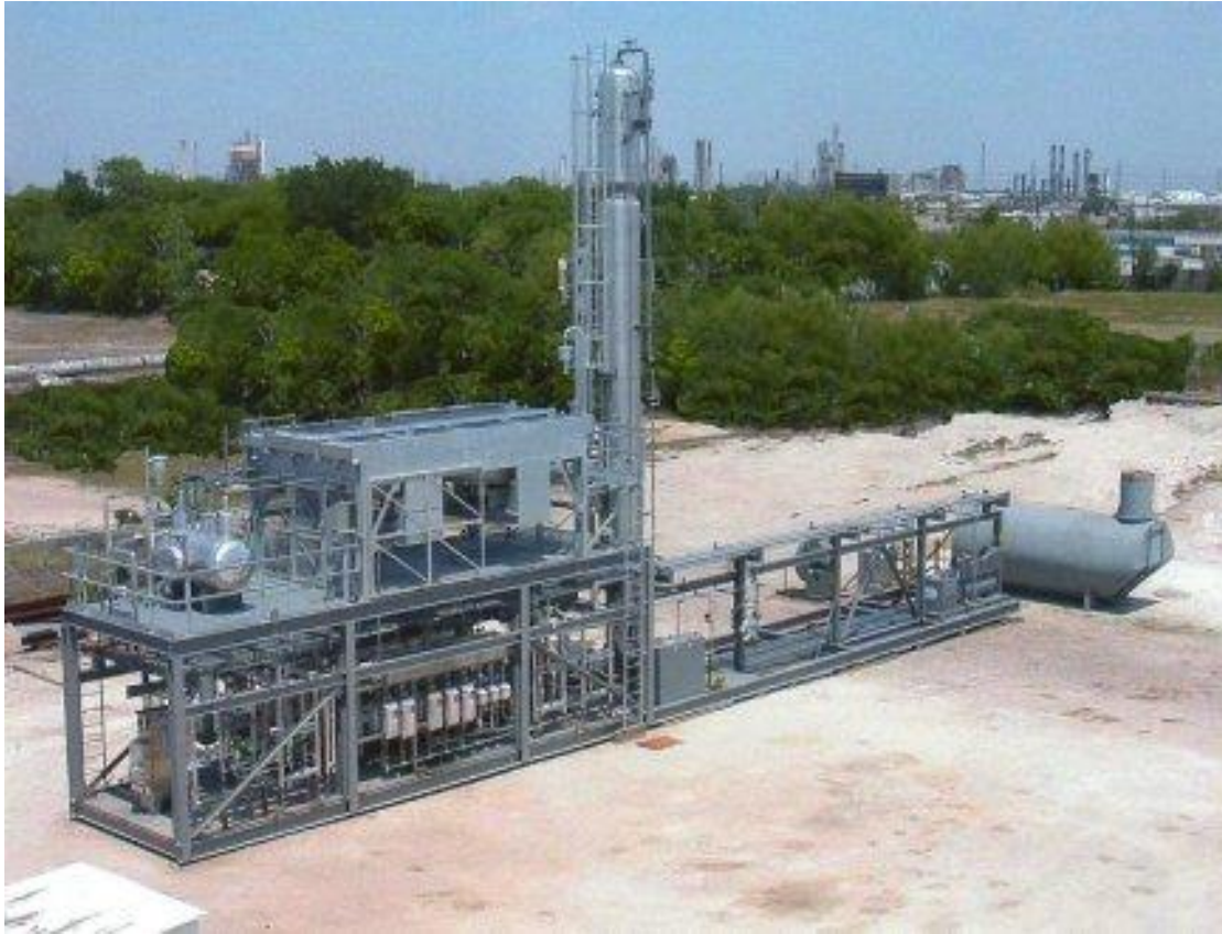
1000BPD Unit being installed
