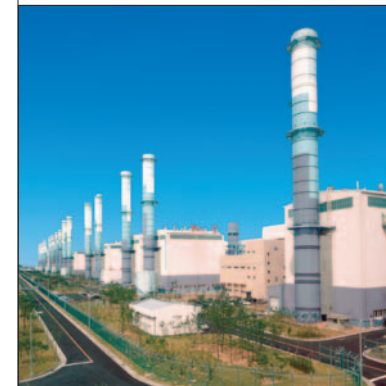
KEPCO's Seoinchon Plant, one of the world's largest combined cycle plants, has operated for more than 40,000 hours in daily start/stop cyclic duty.
