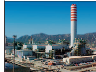
This 550 MW IGCC is located at the Saras oil refinery in Sardinia. The three GE 109E single-shaft combined cycle units have accumulated over 12,000 hours of syngas operation.
