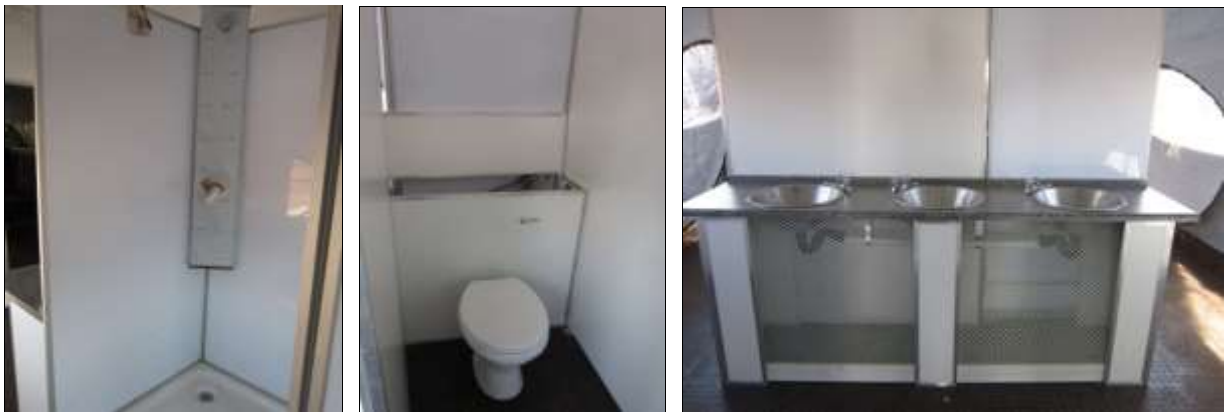
Fig 4: Ablution facilities from left to right: Shower cubicle, toilet and washbasin set.
