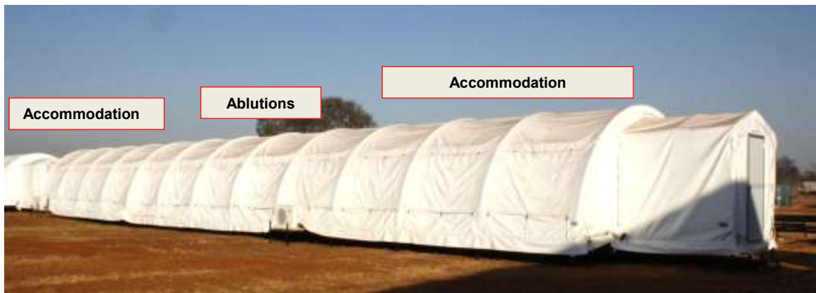
Fig 3: A Warrior based accommodation block consisting of three 4.8m x 9.6m shelters with ablutions in the center.
