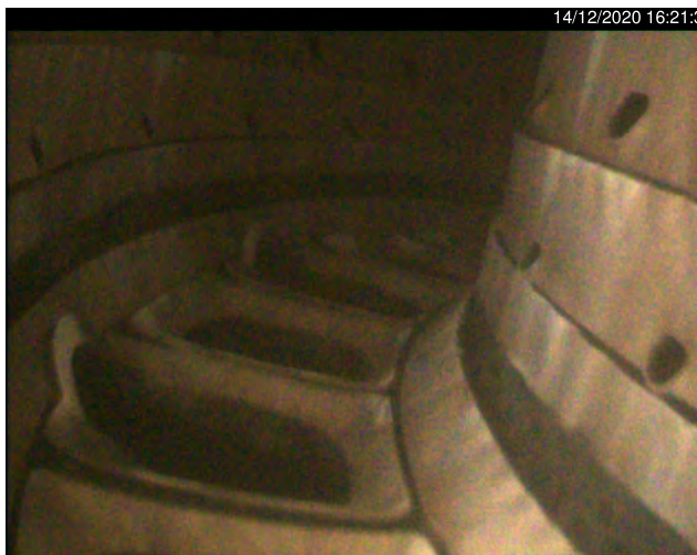
Picture 14: trumpets / splash plates
