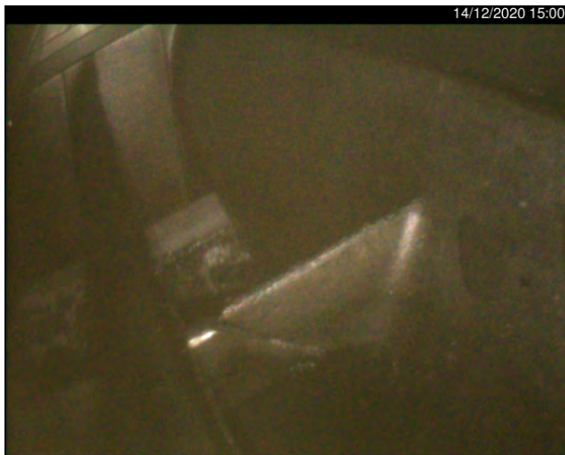
Picture 3: mid span damper
