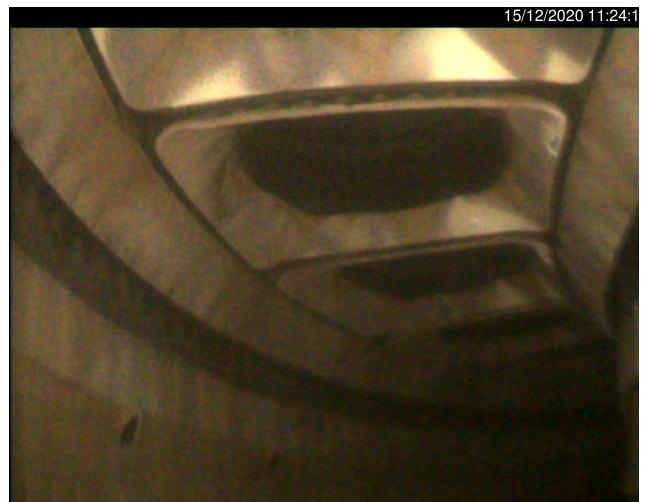
Picture 15: trumpets / splash plates
