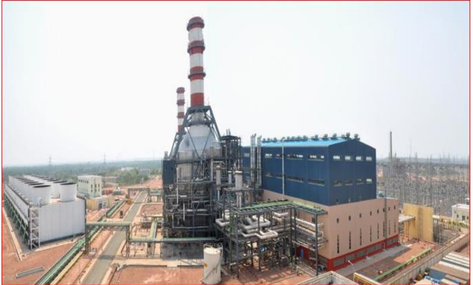
CCPP Power Plant – 2 X 405 MW at ISO cond.
